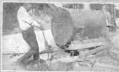
The new ratchet jack device shown above is exceptionally useful in hauling heavy loads with very little man power. It may also be used to raise and lower heavy objects with the use of but one man power. The device is the invention of Mr. E. W. Brantigan.
